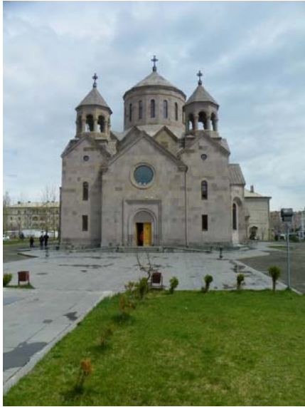
Gyumri, St Hakob Mtsbnatsi church
