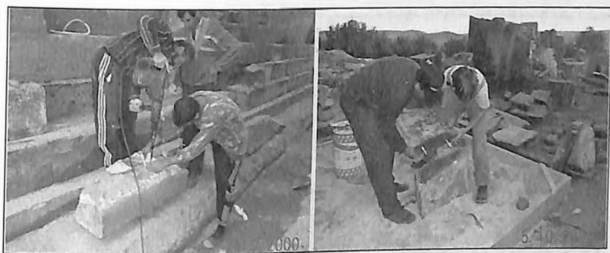
Fig. 3: Big stones are pinned each other
