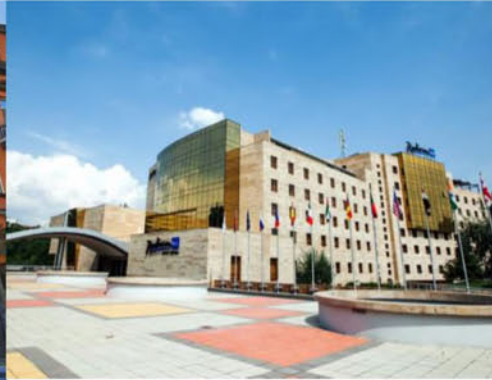
Fig. 2 Radisson Hotel Complex in Yerevan
