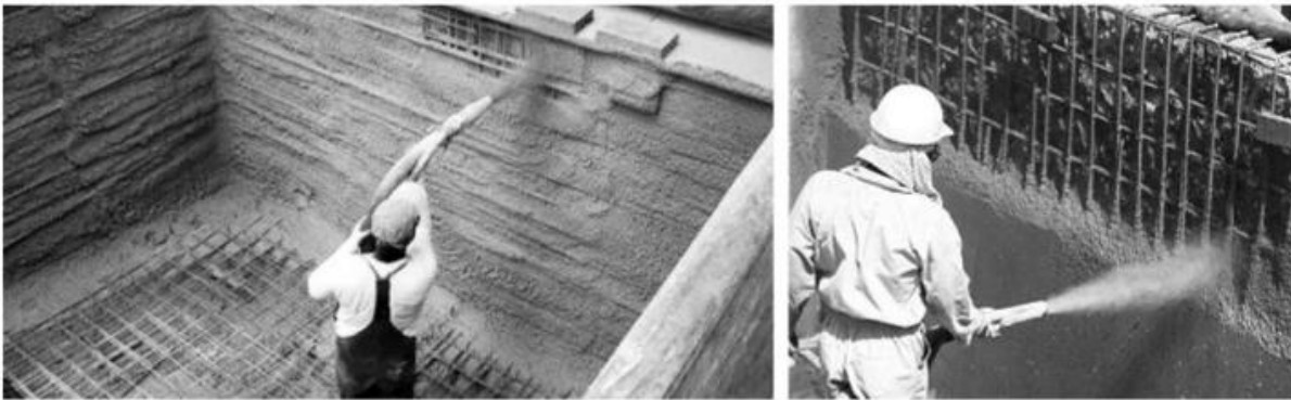
Fig. 3 Shotcreting process
