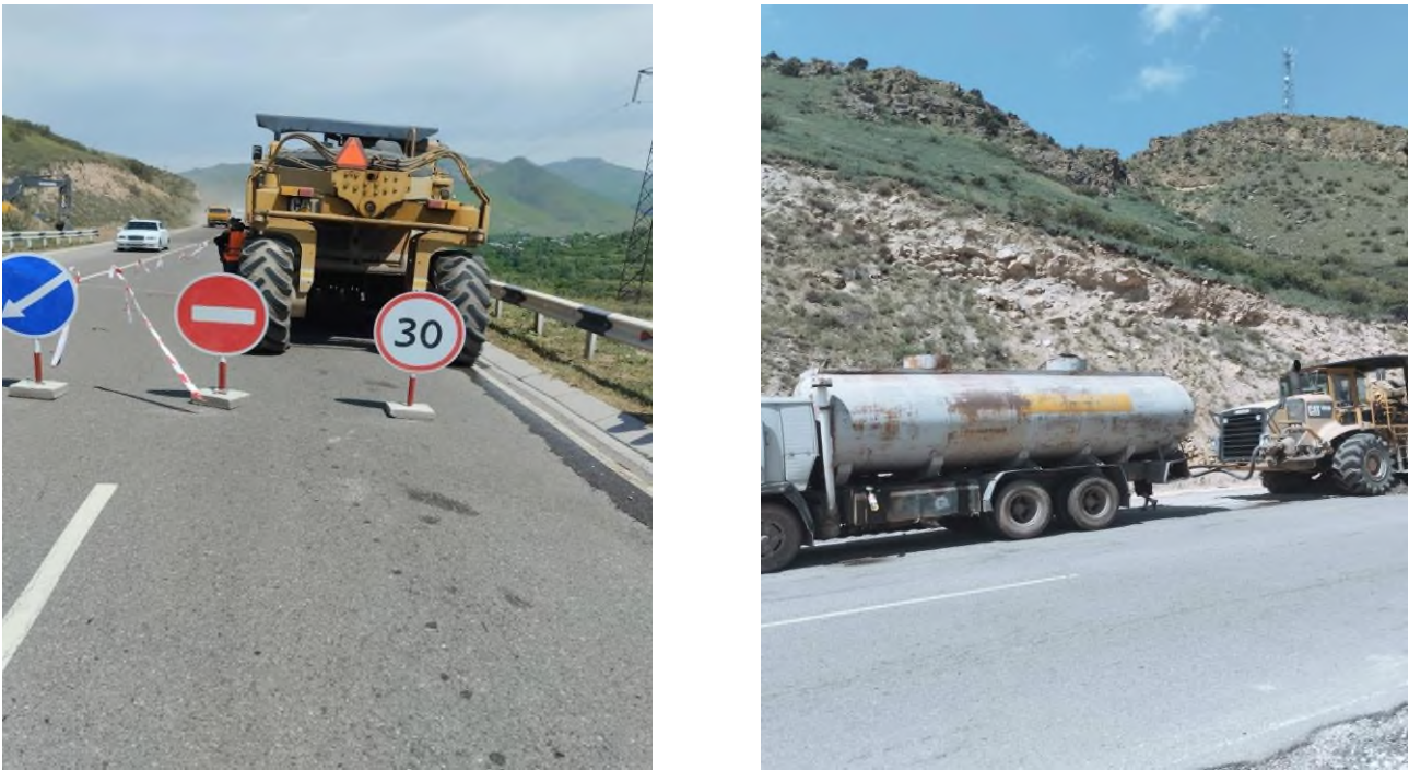
Fig. 1. Section of road under reclamation
