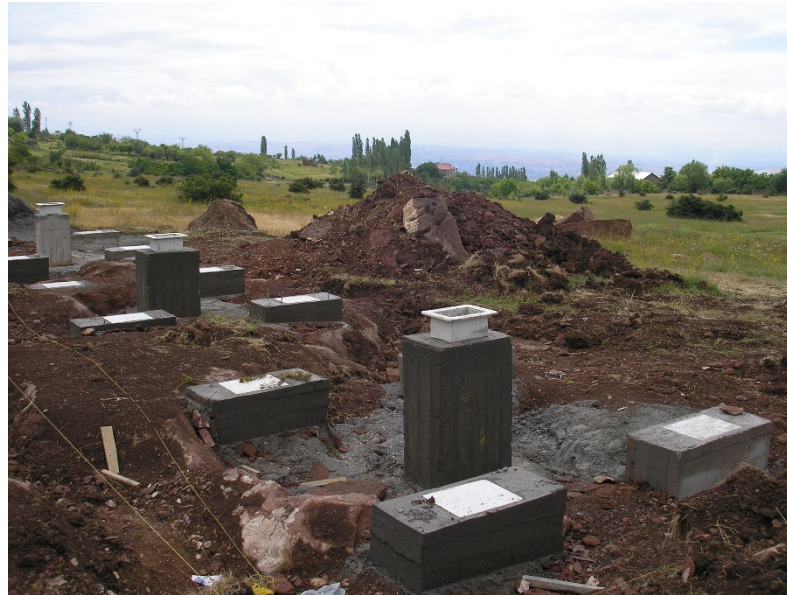
Figure 3. The fundaments of telescopes and containers-domes built at Saravand.
