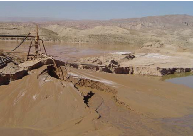
Fig. 4. Tailing deposition in Anguran dam using cycloning method
