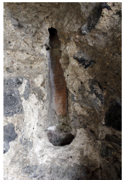
Part of the clay pipe entering the bathroom of the Second bathhouse
