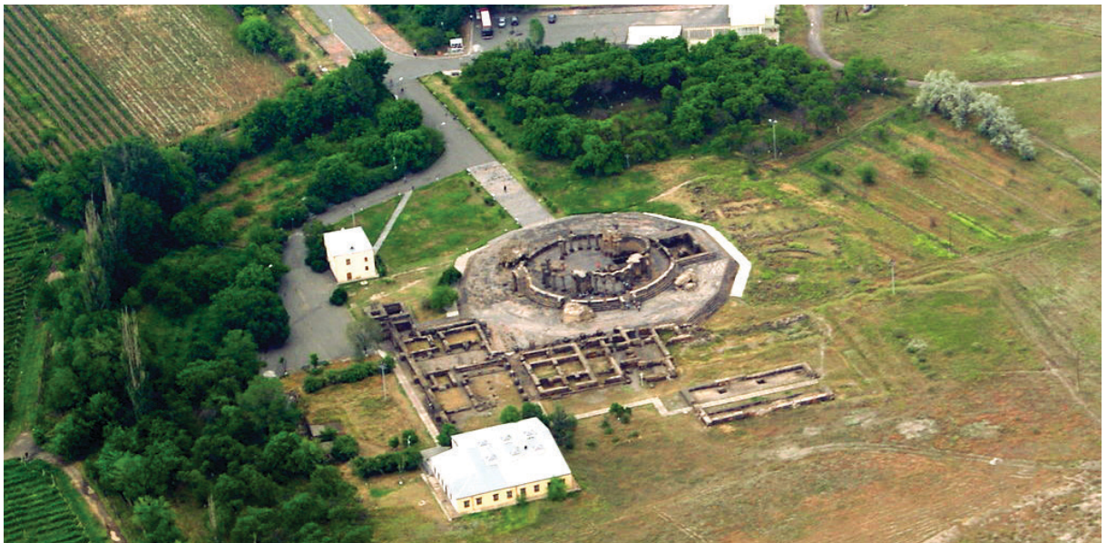
The general view of Zvartnots Temple Complex in 1940-1950s and now
