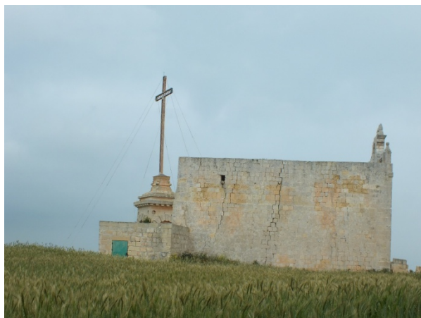
Fig. 1. The wayside church of the Annunciation at Is-Salib tal-Għolja in the parish of Siggiewi showing clear signs of severe structural damages
