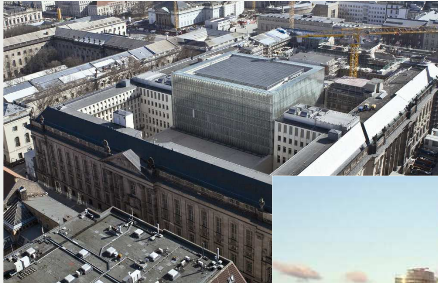
Site on Unter den Linden View from above, new reading room in the center Foto: Axel Gerke, cinemadirekt.com
