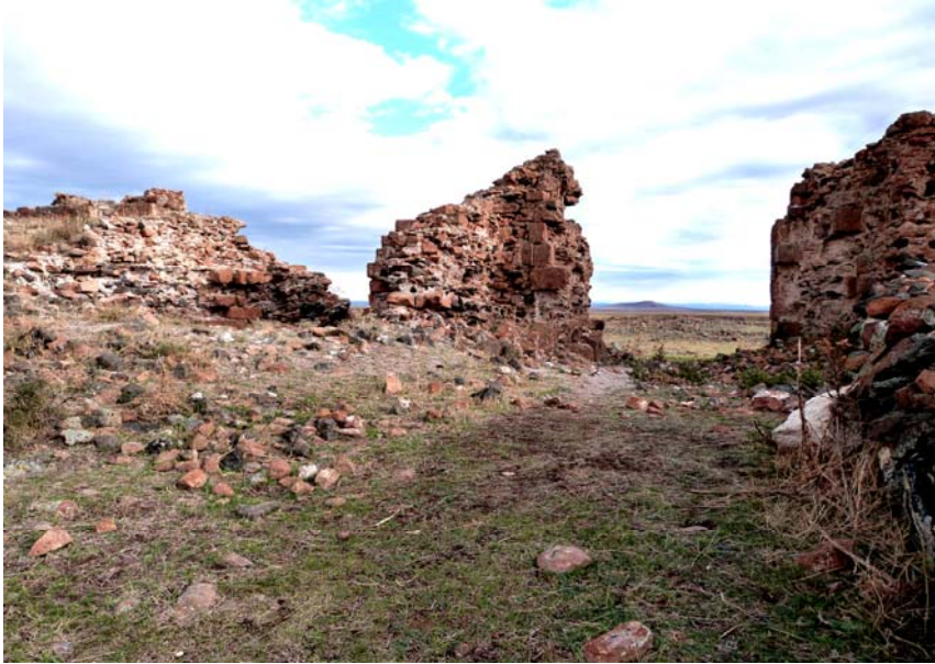
Fig. 9 - Mahasberd, entrance front, gate, outer side.
