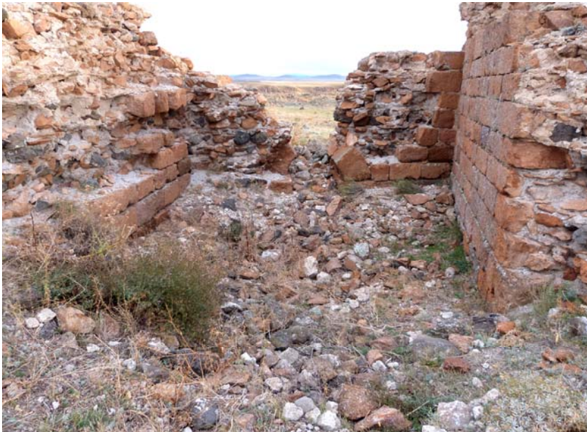
Fig 10 - Mahasberd, entrance front, western tower of the gate
